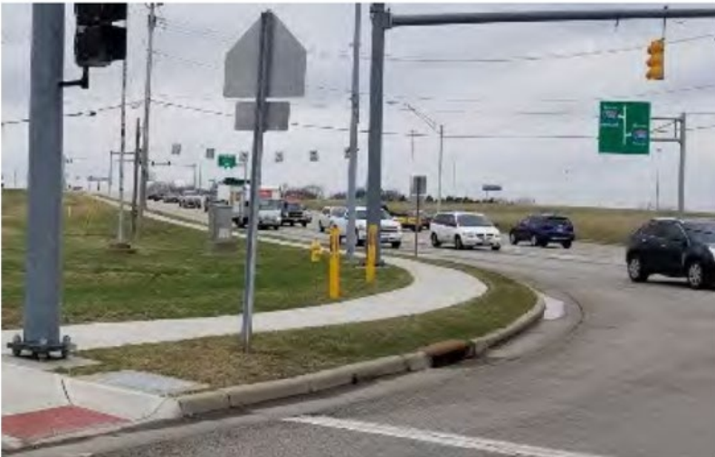
Traffic queues can reach back to the I-280 On-Off Ramp intersection from the Lemoyne Road intersection during peak traffic periods, which causes traffic flow issues
