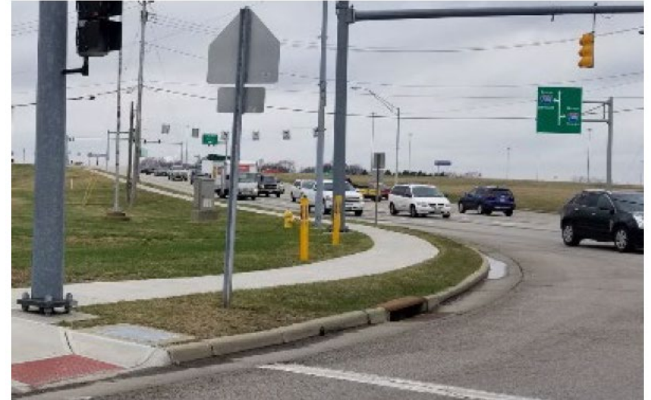
Traffic queues can reach back to the I-280 On-Off Ramp intersection from the Lemoyne Road intersection during peak traffic periods, which causes traffic flow issues
